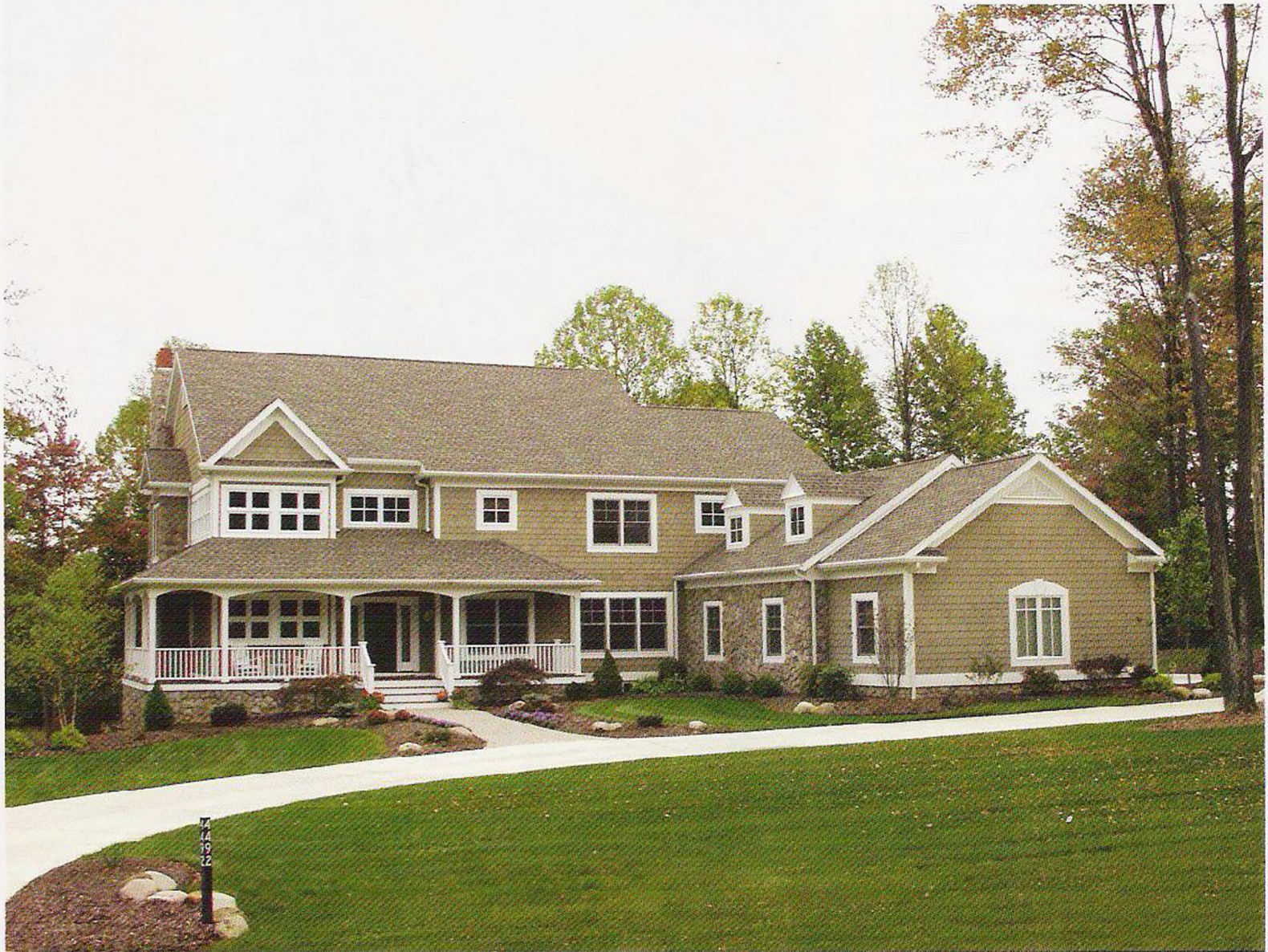
This custom home by Beres Construction won the first place award in the 4,501 square foot to 5,000 square foot category in the HBA's Best Homes Competition in 2002.
